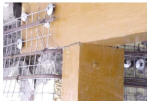
Figure A- 12: continuity at corner behind wood post obstruction
