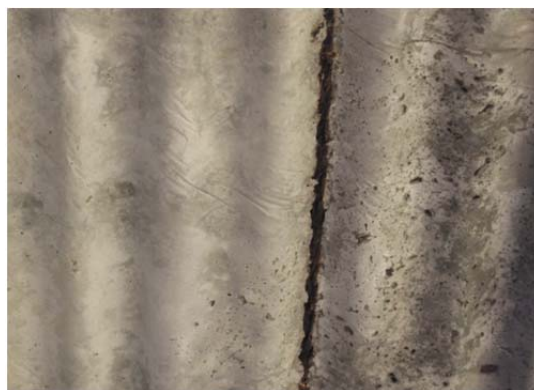
Rebar exposed in RCC slab
