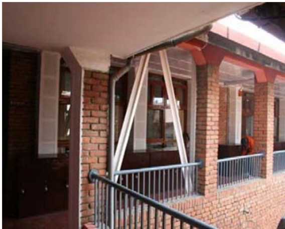
Fig. A.I.9 Retrofitting by Diagonal Steel Bracing
