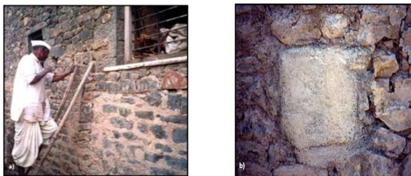
Figure 4.43 Examples of through-stone installation in Maharashtra, India: a) removing stone from the existing wall, and b) surface of a through-stone covered with a plaster (Source: UNDP, UNESCO & GOI, 2007)
