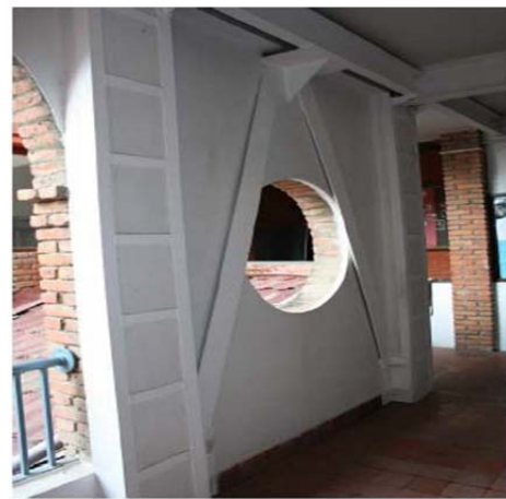
Fig. A.I.9 Retrofitting by Diagonal Steel Bracing
