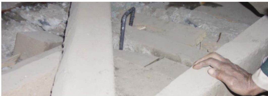
Figure A- 17: Anchoring vertical bars over wall-plate at attic deck
