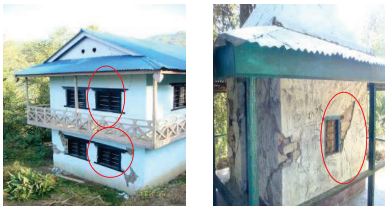
Figure 2.24 Some examples of Cracks at opening
