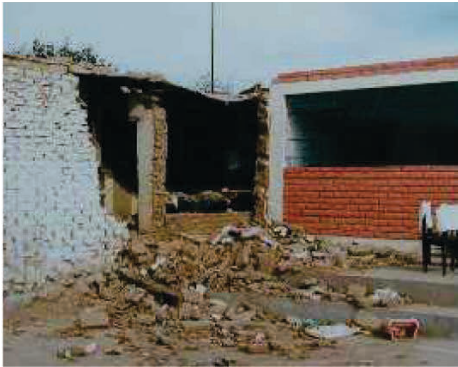
Figure 2.7 Out-of-plane wall collapse – 1996 Nazca earthquake, Peru (Source: Report #52 in EERI/ IAEE World Housing Encyclopedia)
