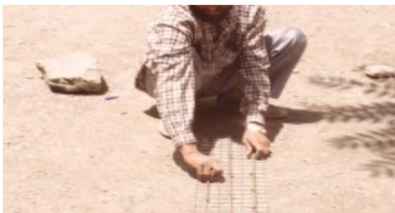
Figure A- 7: Preparing WWM with 6 mm rebars
