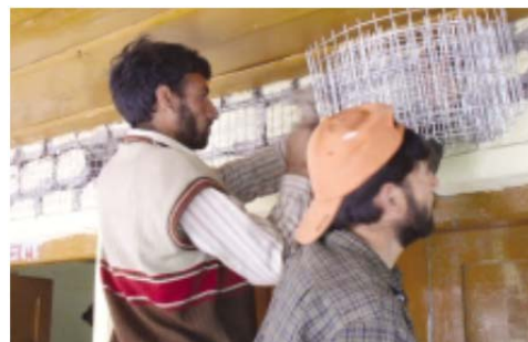
Figure A- 8: Installing WW mesh from a roll
