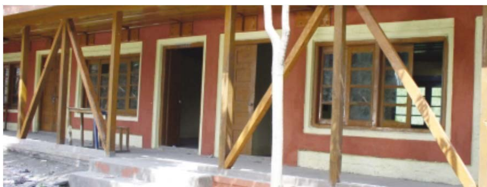
Figure A- 20: Retrofitted building with belts, roof anchoring and diagonal timber bracings
