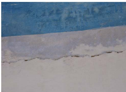
Cracks at slab & wall connection
