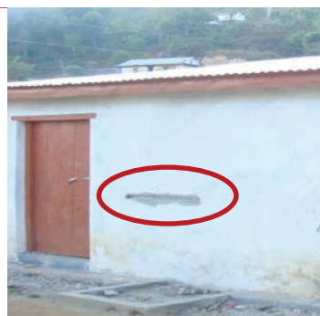
Figure 2.14 Mid-height Crack (Photo: CoRD)
