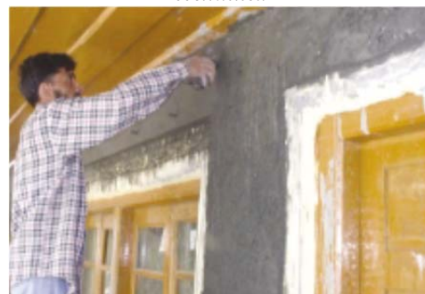
Figure A- 14: plying cement-sand plaster
