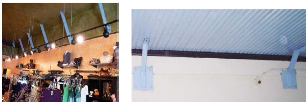
Figure 4.31 Roof to wall connection
