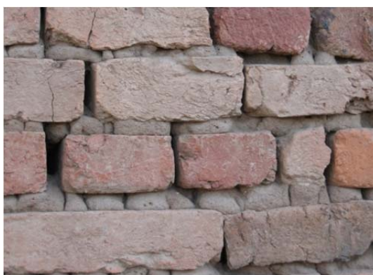
Void between masonry units
