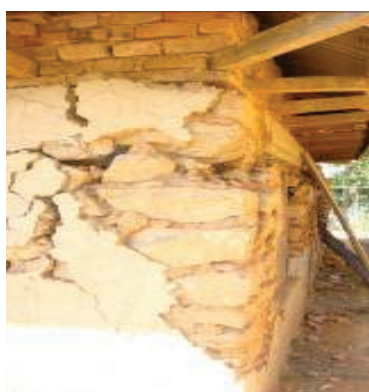
Figure 2.18 Some other examples of corner damages (Source: CoRD)
