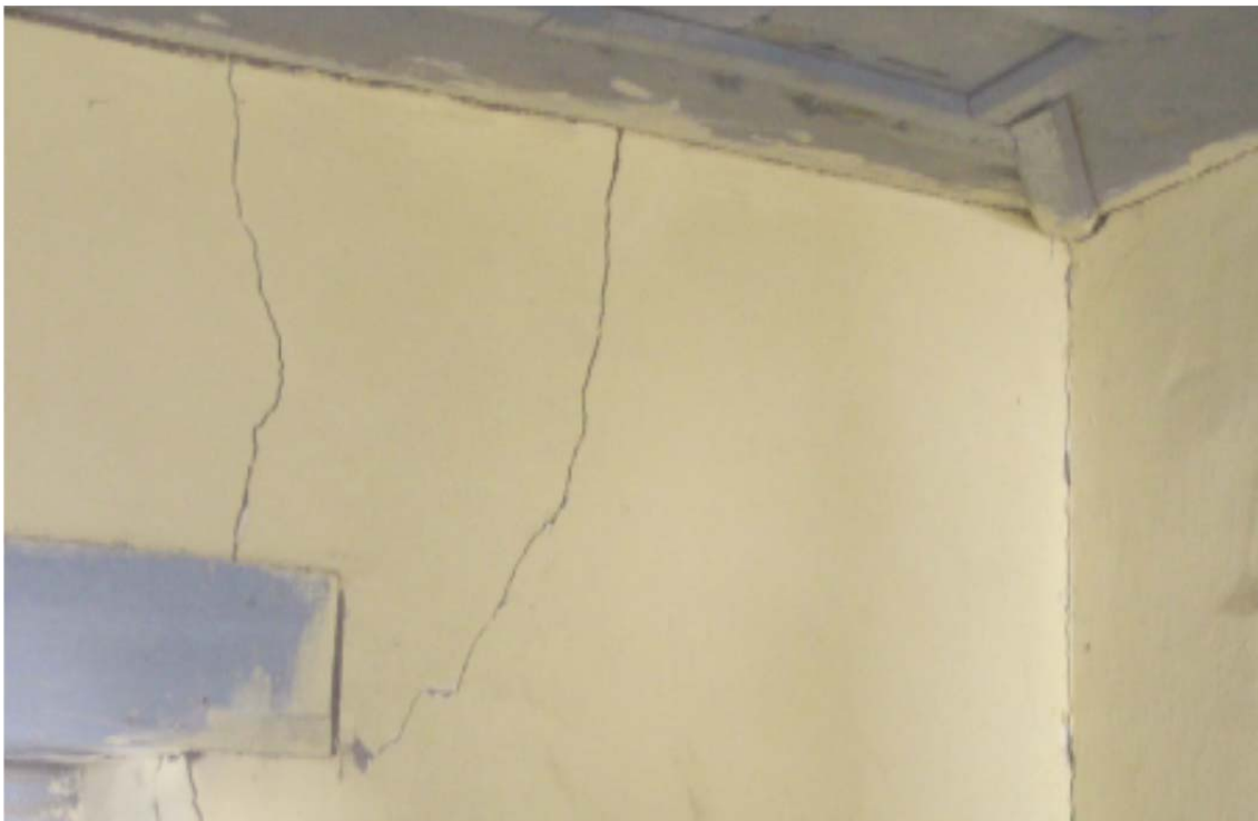
Figure A- 3: Typical cracking in corners and at corners of opening such as windows
