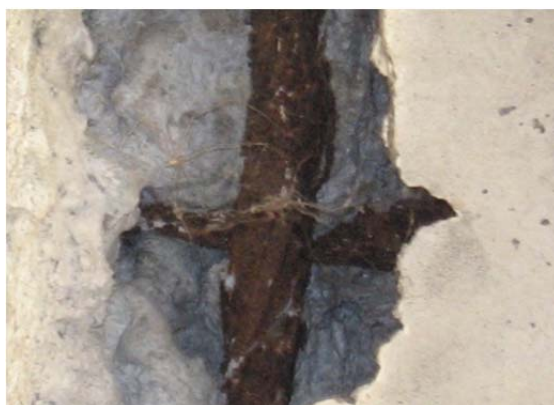
Exposed reinforcement
