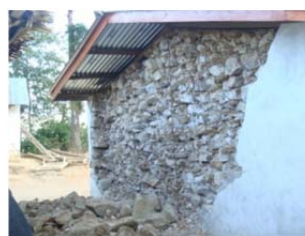
Figure 4.37 Delamination
