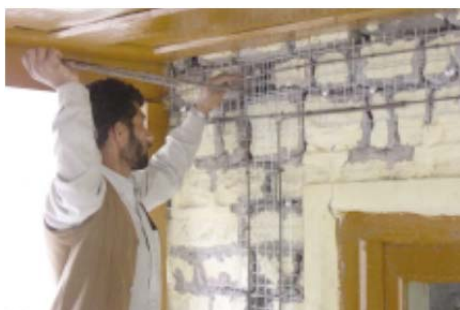
Figure A- 11: Inserting dowel for belt to belt connection at corner
