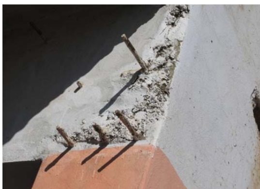
Rebar exposed at beam ends
