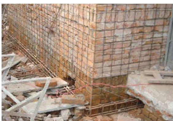
Fig A.I.4(b) Erection of Reinforcement for wall
