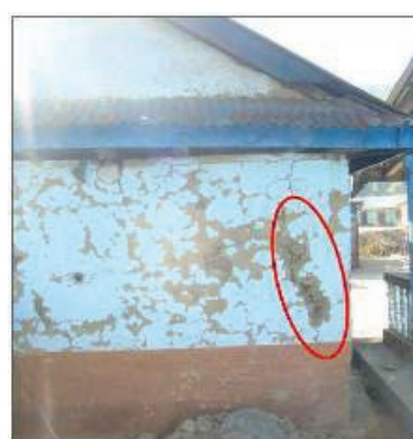
Figure 2.18 Some other examples of corner damages (Source: CoRD)
