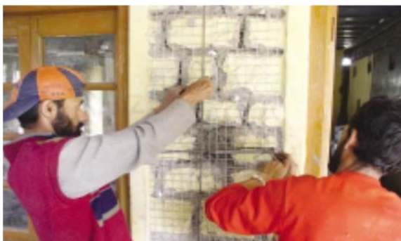
Figure A- 9: Tying encasement reinforcement to shear connector dowel
