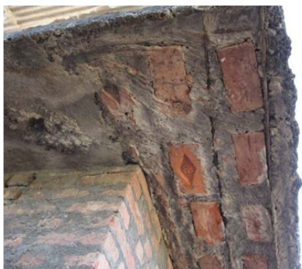
Rebar exposed in RBC slab
