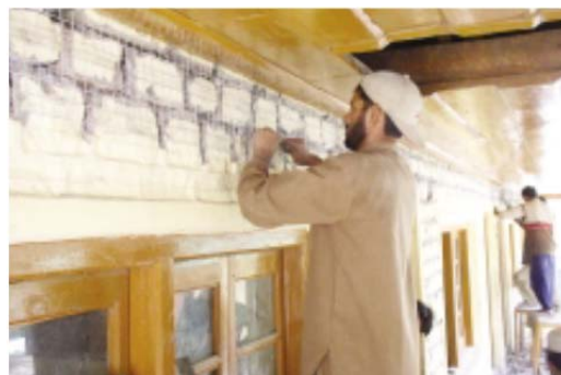
Figure A- 10: Installing belt reinforcement
